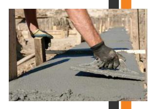
All concrete must possess an open surface texture with all curing compound and sealers removed. All areas should be pre-wetted to reduce moister loss. Do not place product on standing water.
